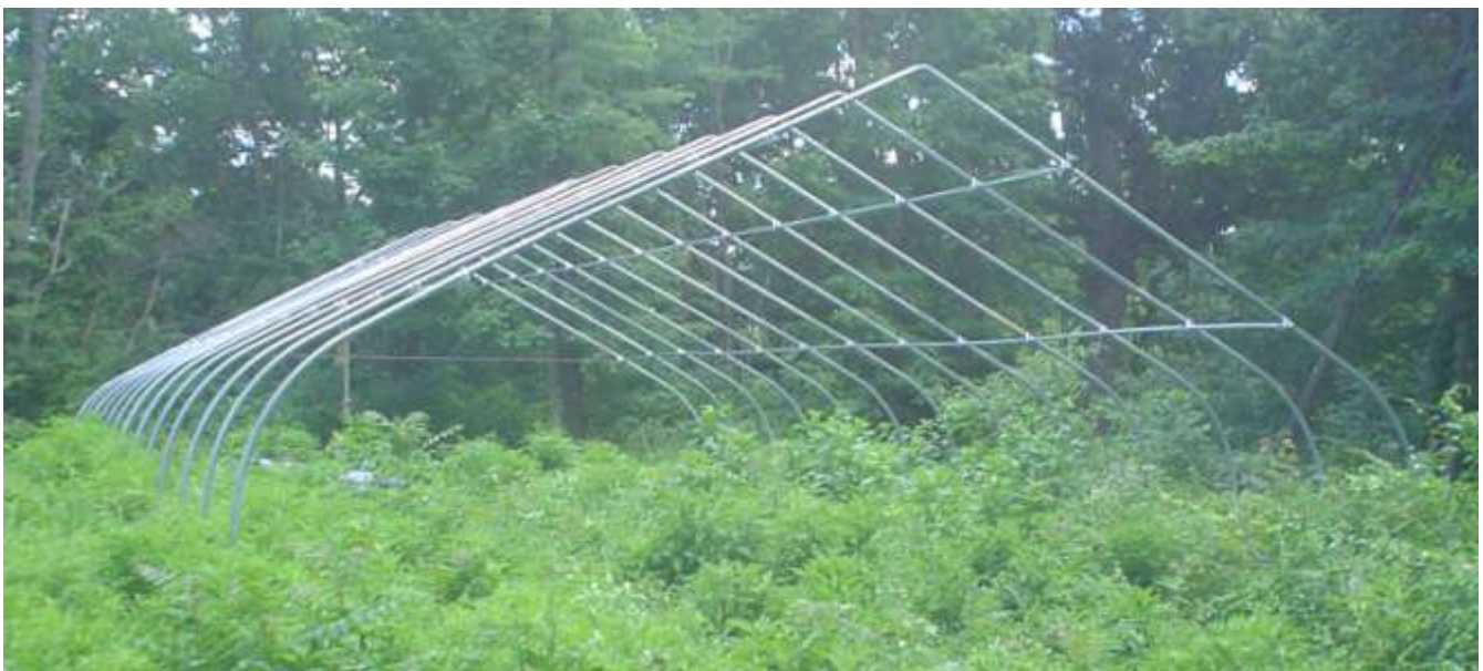
A New Hoop House Under Construction
